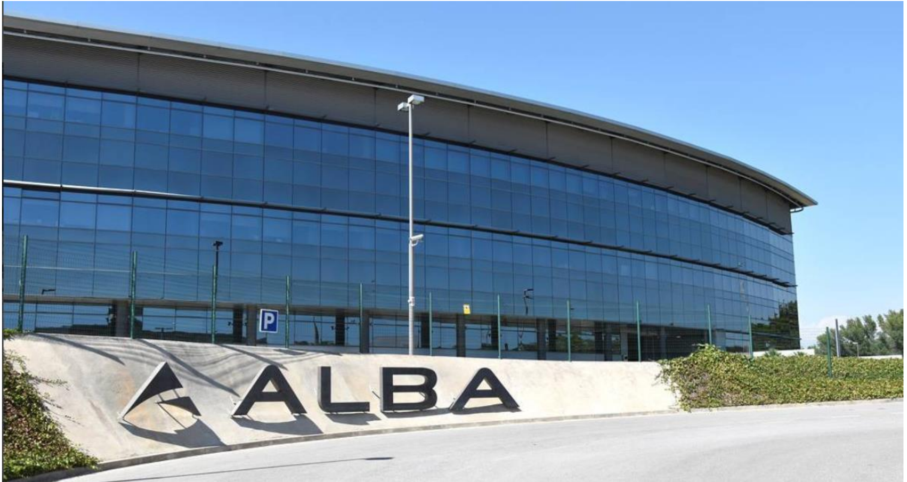
ALBA Industrial Office
